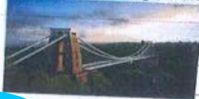
Clifton Suspension Bridge, Bristol
